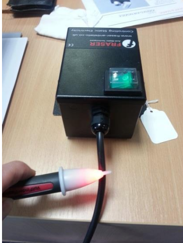
Figure 2. Volt stick verifying that mains supply is good.
